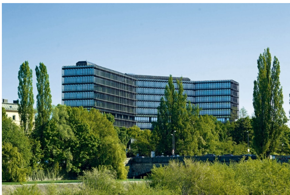
Figure 15 – OEB Munich, bâtiment Isar
